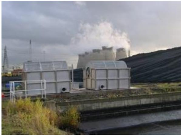
The coal stockpile fines were accumulating rapidly and creating potential release issues due to overflowing. Two rotary drum screens were installed to recover the fines for reuse and alleviate the problem of rapid build up on site.
