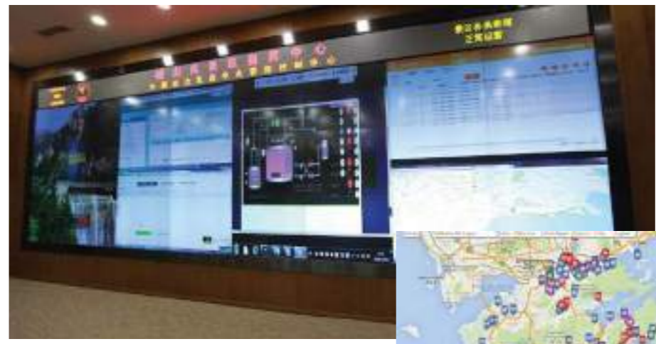
Remote monitoring each bio-toilet system
